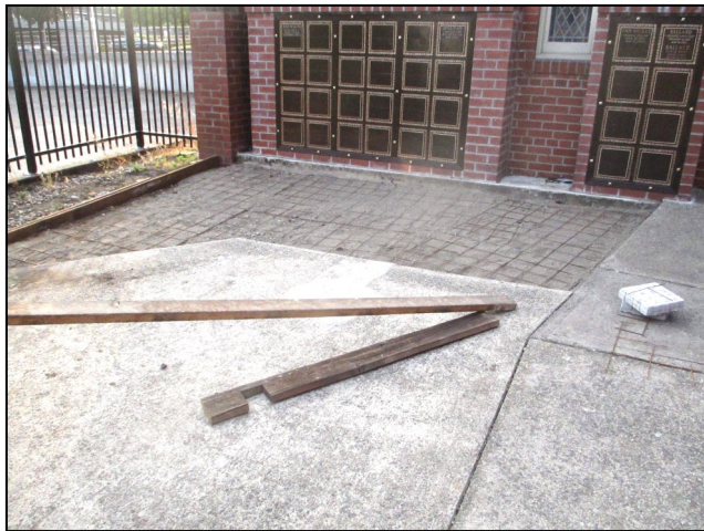
Above: area to be filled with concrete showing the rebar matting.
