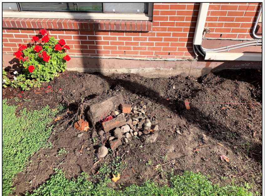
Charles Van Sickle is digging up rocks, concrete, and clay to prepare for planting trees in front of the office.
