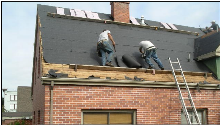
The Rectory has been roofed with one-inch tongue and groove solid sheathing. These shots were taken on July 21 by Bill Riley.
